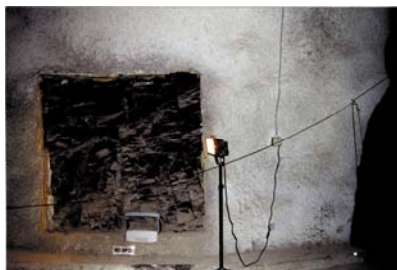
Contour destrengthening behind shotcrete liner
