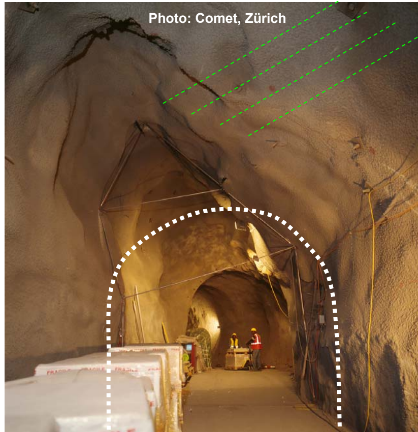
Bedding plane failure
