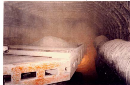
Backfilling Slinger Truck in a Disposal Drift
