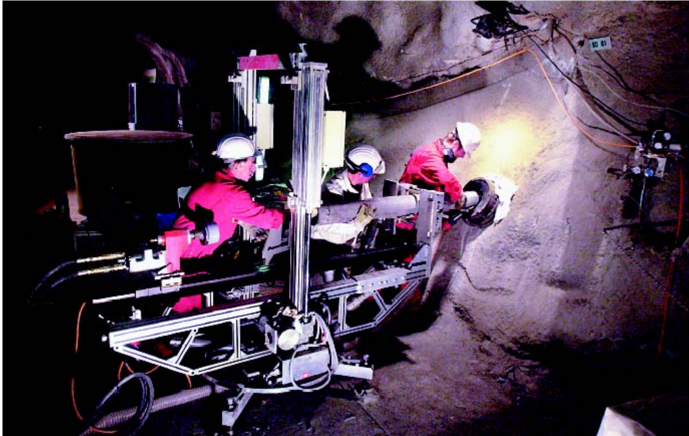
Installation of the overcoring drilling rod
