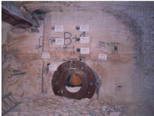
Backfill sampling around the central heater after dismantling
